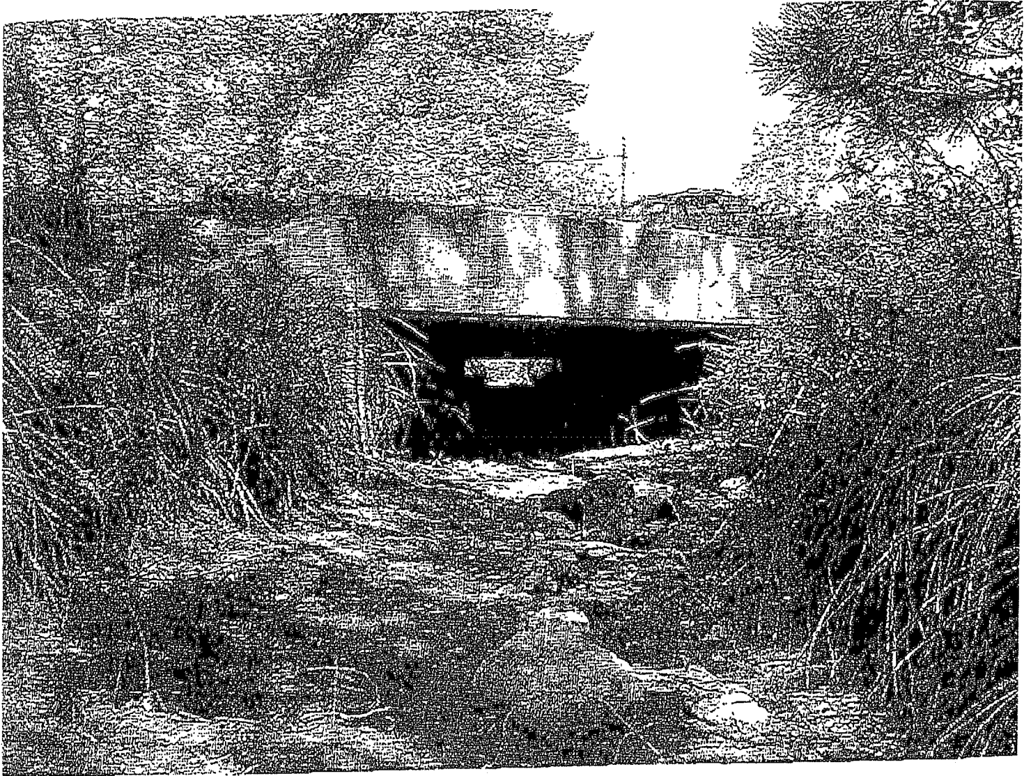
Enterprise Ditch crossing at Arapahoe Road Boulder County, CO - upstream face
